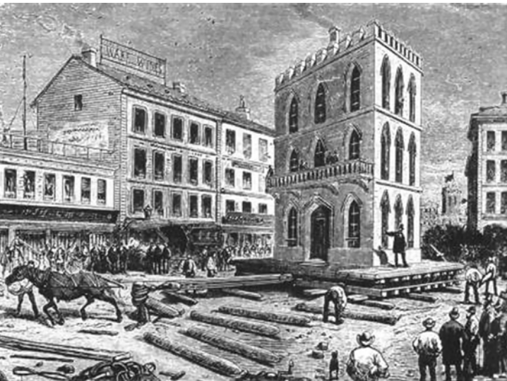
Fig. 26 Moving a Building in Chicago. 1877.
