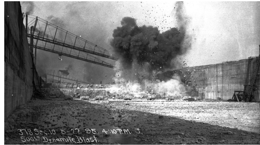
Fig. 22 Dynamite Blasting Through Bedrock During the Construction of the Chicago Sanitary and Ship Canal. May 22, 1895.
