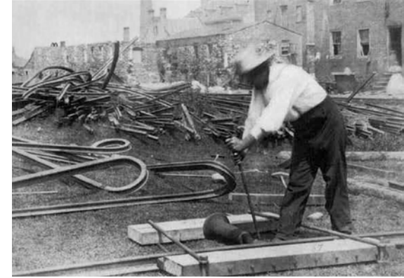
Fig. 36 Railroad Construction Worker Straightens Track for the Union During the Civil War. 1862 – 63.
