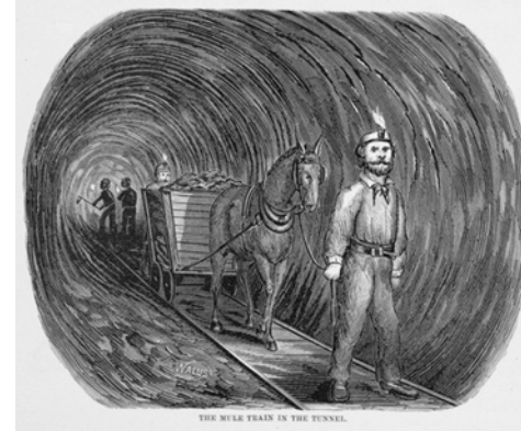
Fig. 21 The Mule Train in the Tunnel. 1874.
